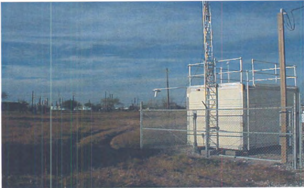
Site (3) Huisache CAMS 98 (TCEQ Existing - looking west WNW)
