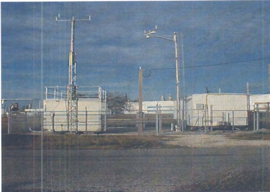
Site (3) Huisache CAMS 98 (TCEQ existing - looking N)
