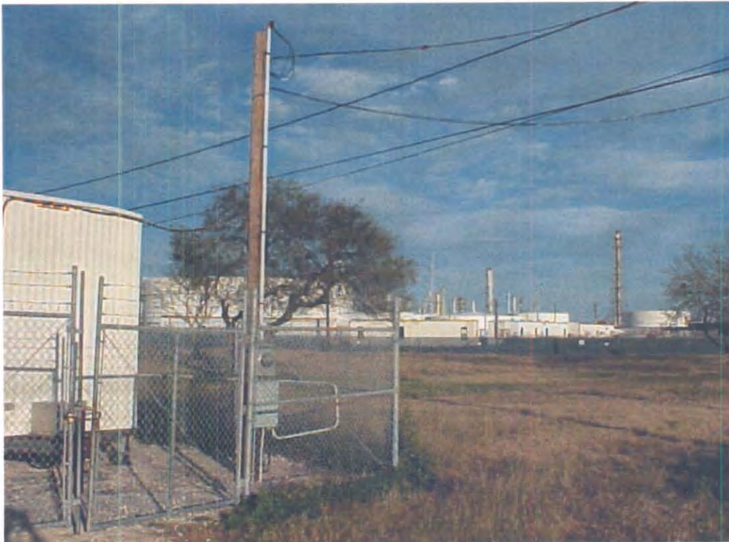
Site (3) Huisache CAMS 98 (TCEQ Existing - looking ENE)
