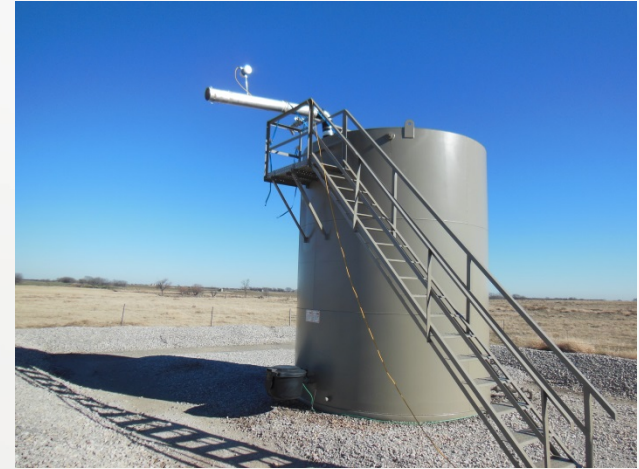
Measurement Connection to Tank (Gas Well Unloading)
