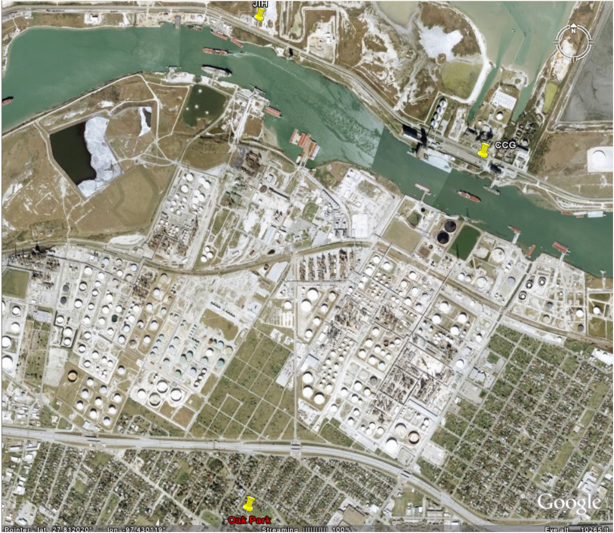
Figure A.7-19. Detail map of the Port Grain monitoring station and surrounding area. The J. I. Hailey and Port Grain monitoring stations are on the north bank of the Ship Channel in the upper middle and upper right corners, respectively. Note a number of industrial areas associated with various facilities (e.g., refer to Figure A.6-1) are located in the nearby area, including various dry and/or liquid bulk loading/unloading docks along the Ship Channel.
